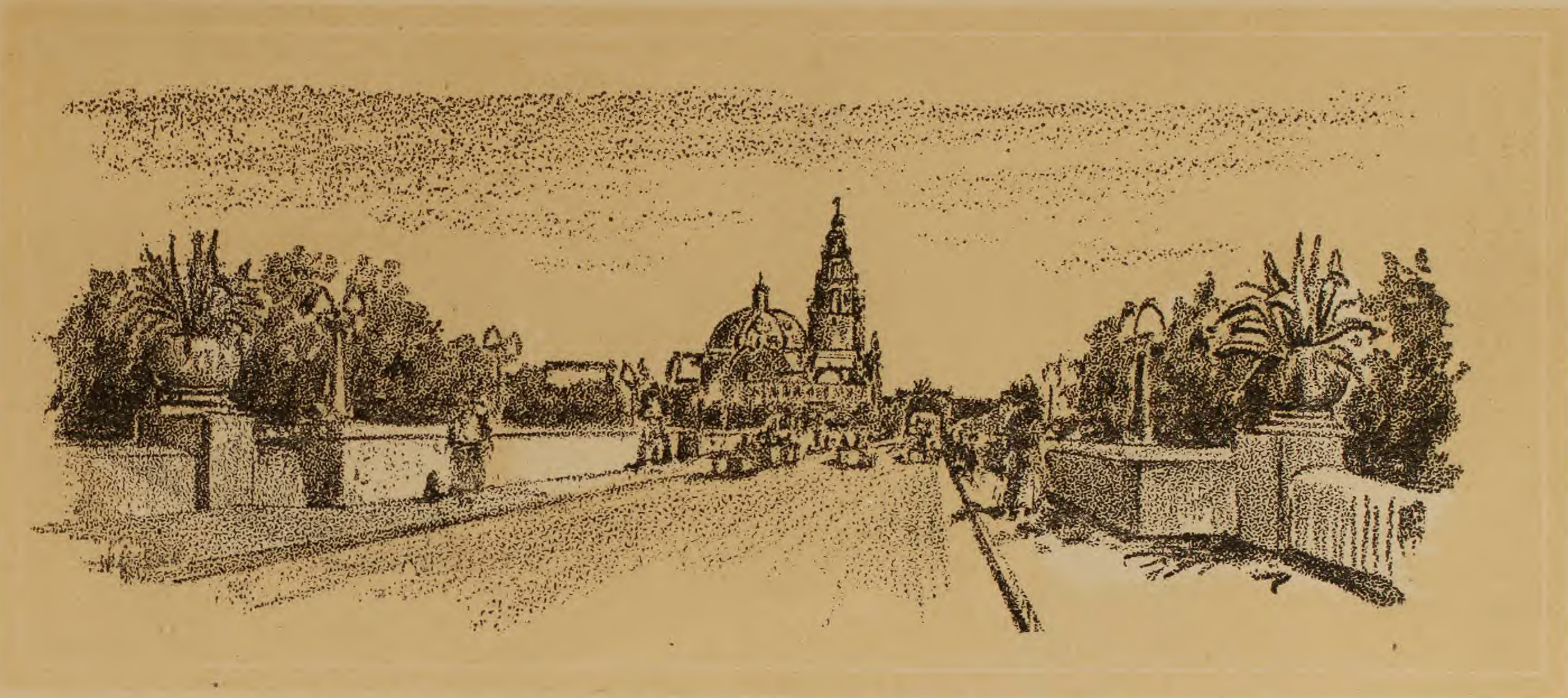
ACROSS "EL PUENTE CABRILLO" LOOKING EAST TOWARD THE ARCH OF THE OCEAN
